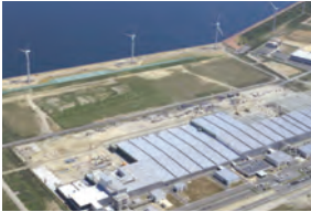
Kitakyushu Plant in Japan
