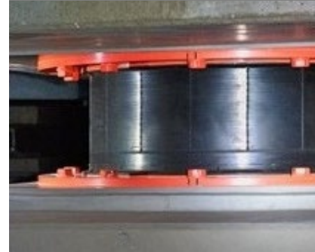
Seismic Isolation Bearings
